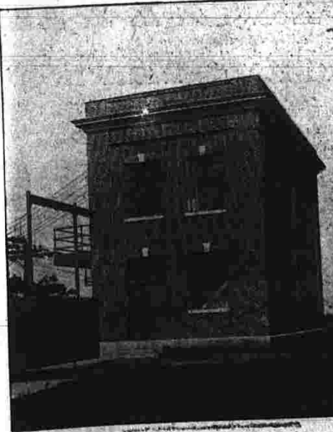
Exterior View of Station
